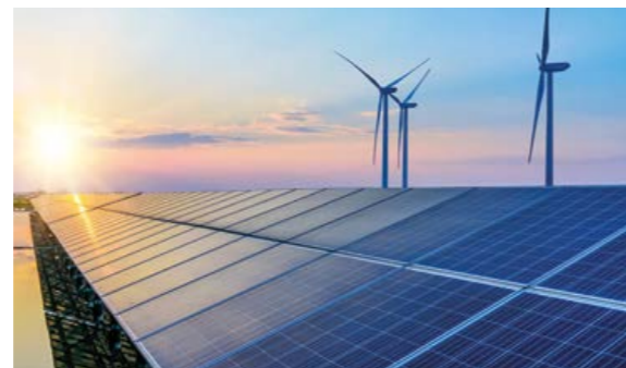
Solar panels on plant Avelgem
